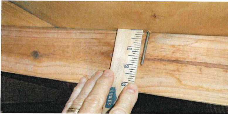
8d nails verified
