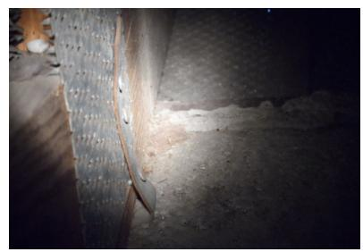
Single strap (clip) with at least 3 nails into the truss
