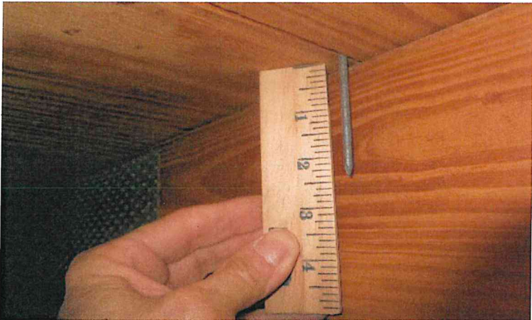
8d nails verified
