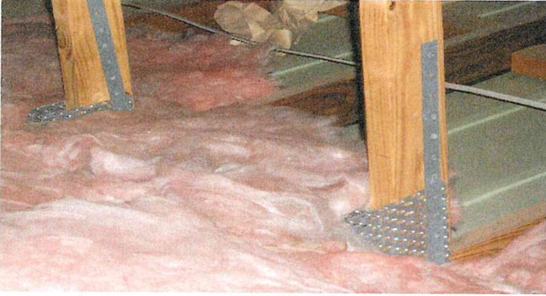
Single strap (clip) with at least 3 nails into the truss
