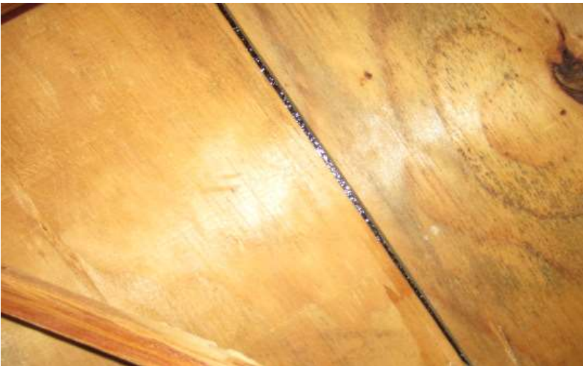
SWR installed under the tile
