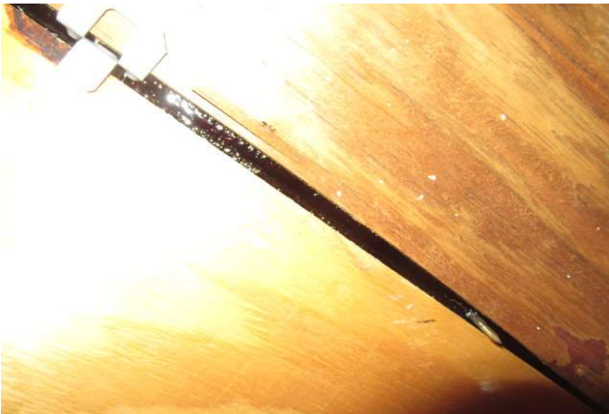
SWR installed under the tile
