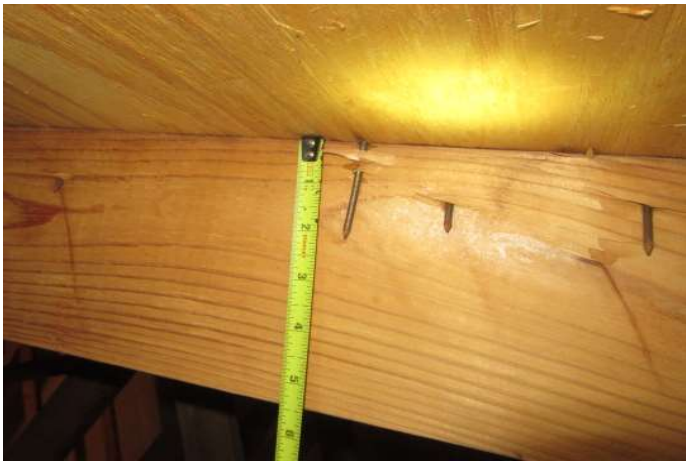
8d nails verified
